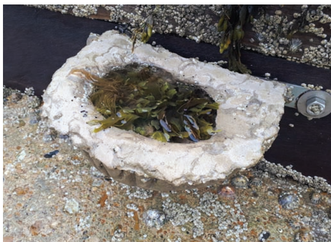
Compton style Vertipools on a wooden groyne on the Science Beach at Sandown, UK
